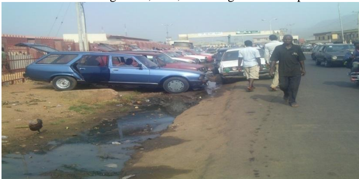
Plate1: Dilapidated Road Landscape at New Market Motor Park, Lokoja
